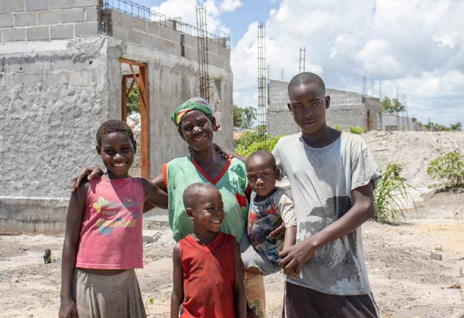
Vitória Poito with four of her seven children in front of her new house under construction one of the many resilient single-family houses being built in Mutua neighborhood after the passage of Cyclone Idai in 2019, as part of the UNDP's Mozambique Recovery Facility. Sofala Province, March 2021. © UNDP Mozambique/Brenda Hada
